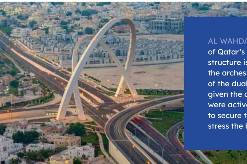
**AL WAHDA ARCHES** dominate the blue-sky landscape of Qatar's capital, DOHA. Standing 100m tall, the structure is constructed of 9,000 tonnes of steel, while the arches are clad with Limra Limestone. Construction of the dual arches presented an engineering challenge given the angles and size of the project. Macalloy were actively involved supplying 1030 BARS in 75MM to secure the foundations and Hydraulic Jack units to stress the bars.
